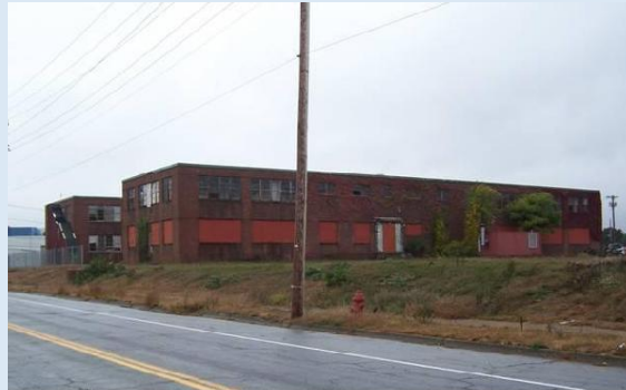
These old buildings are slated to be demolished.
